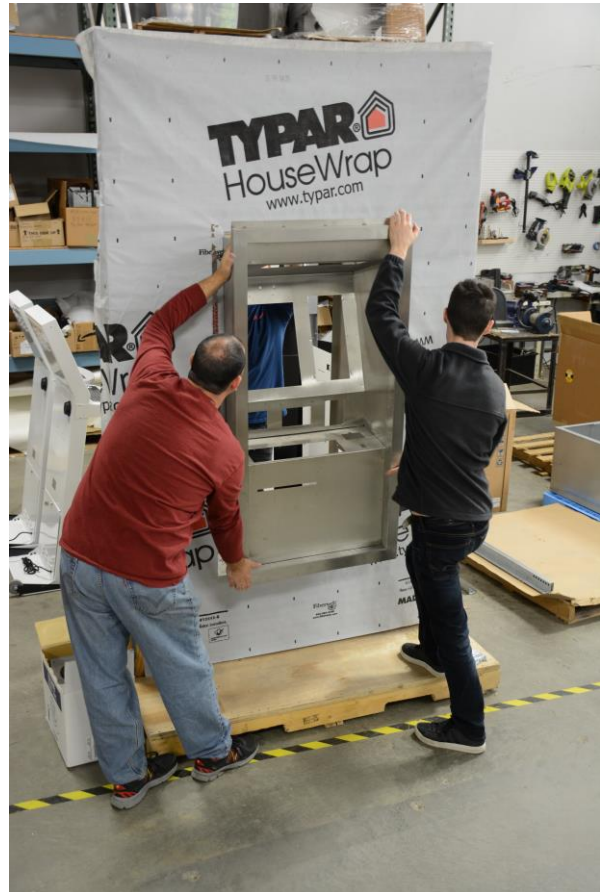
2. Kiosk Assembly Being Pushed into Wall
