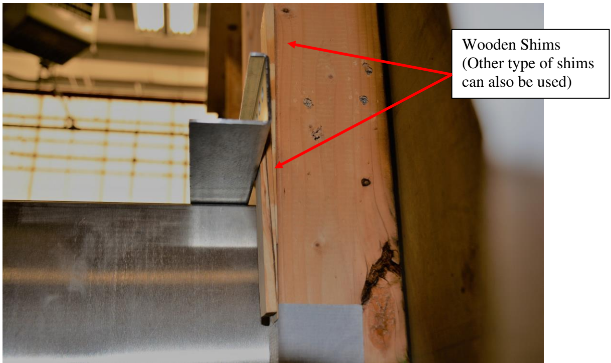
Shims Between Bracket and Wall
