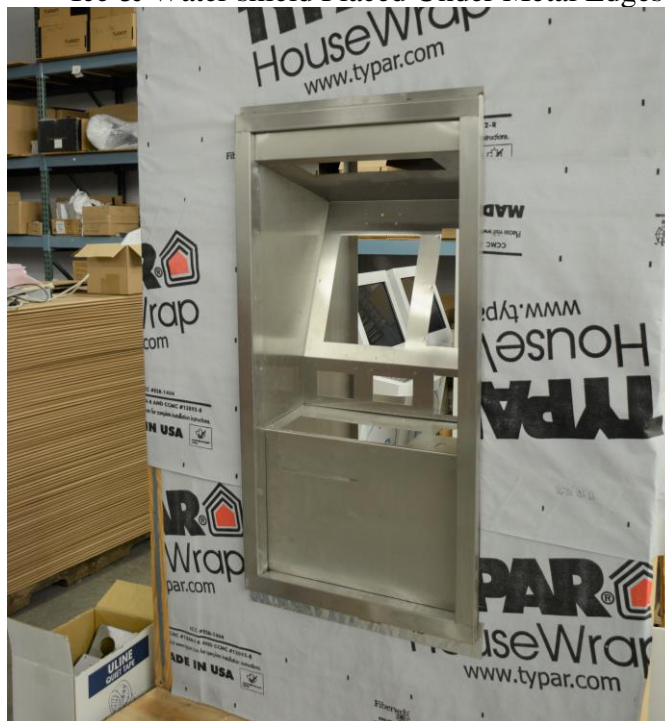
Kiosk Fully Pushed into Wall
