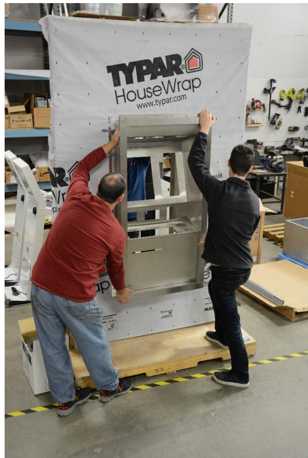
2. Kiosk Assembly Being Pushed into Wall
