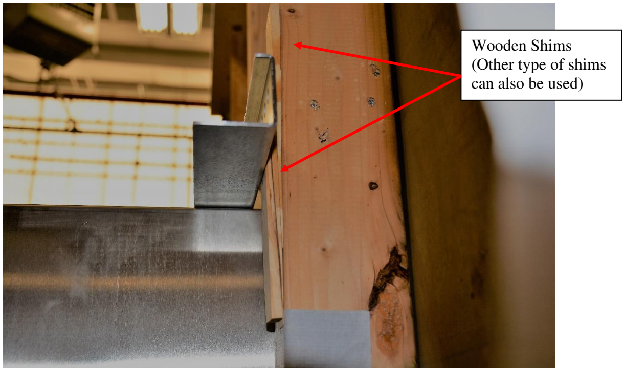
Shims Between Bracket and Wall
